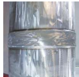
Completed overlay sanding on a pressuriser nozzle
